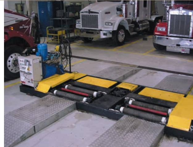
Low profile VIS-Check conveniently mounts on the floor of a conventional service bay.
